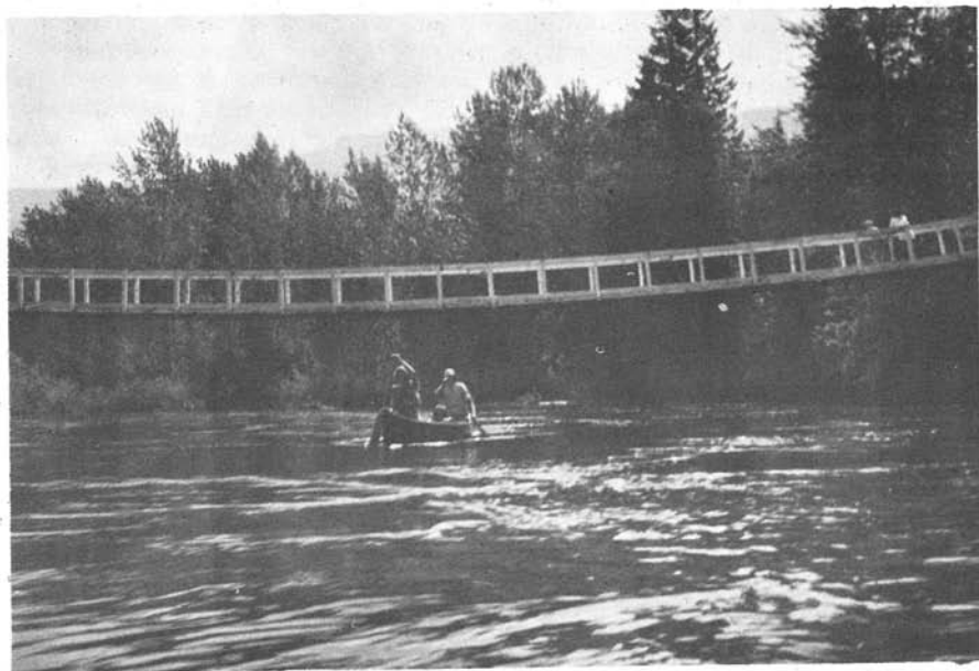
Suspension bridge on Eagle River.
