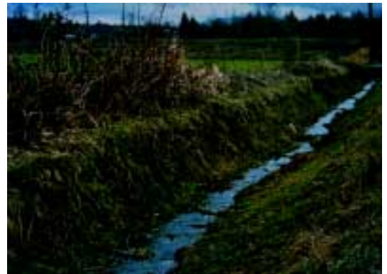
A well designed drainage plan will include ditches designed to accommodate flows without the requirement to clean frequently.
