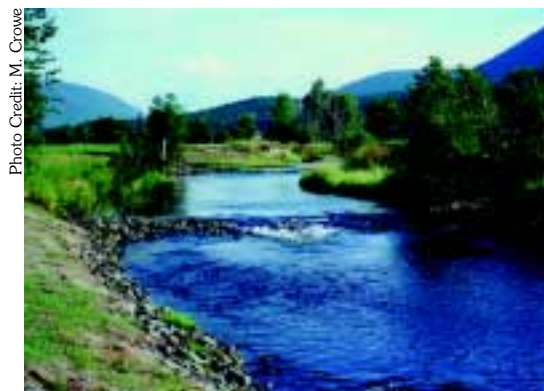
Where streams have been severely damaged, restoration projects are required to restore habitat. This photo shows stone placed to protect the banks and create riffles and pools in the stream.
