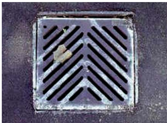
Figure 10: Drain (Catch Basin)
